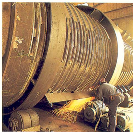
Calcined coke cooler
